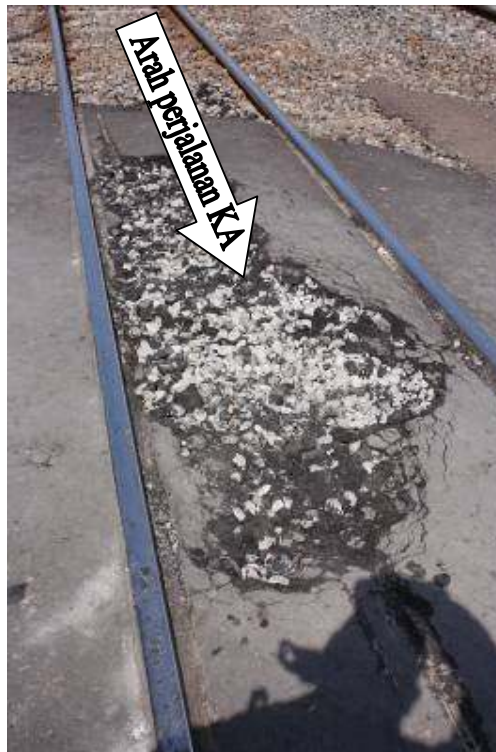
Gambar 19. Bekas gerusan tread brake housing di aspal perlintasan JPL 324
