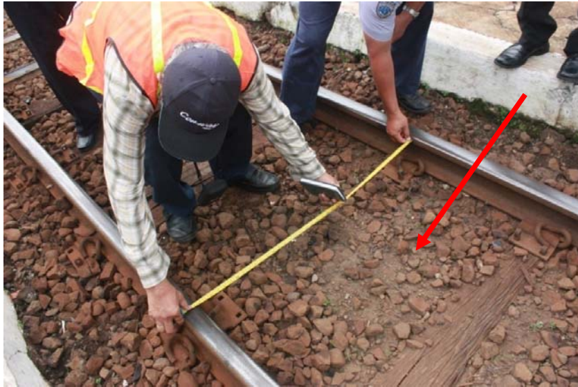
Gambar 12. Ballast kurang
