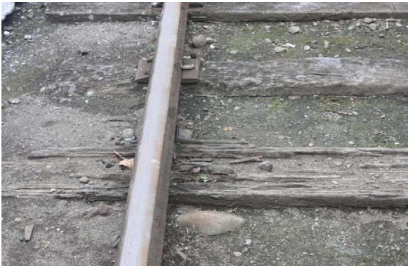
Gambar 13. Ballast kurang
