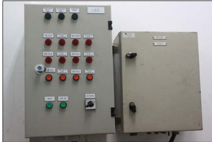
Gambar 13. Link Breaking Device
