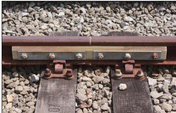
Gambar 15. Insulated Rail Joint
