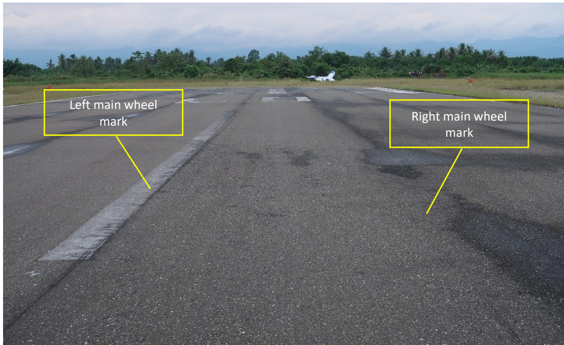
Figure 6: Tire marks found on the runway
