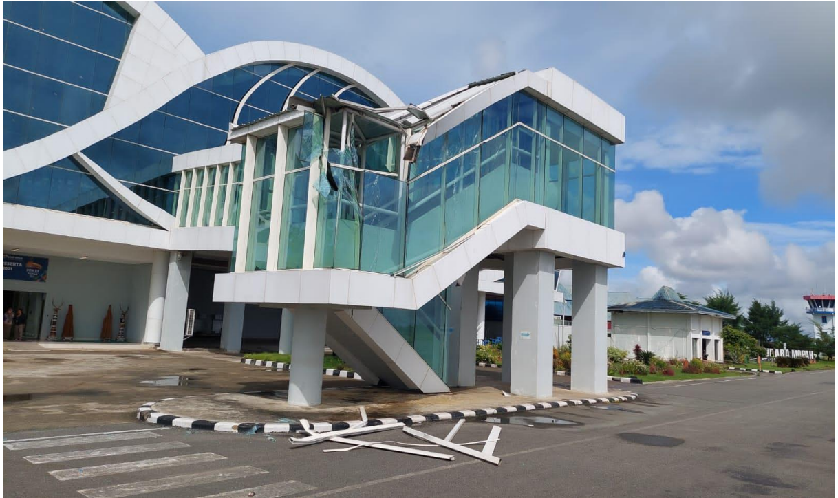
Figure 8: The damaged airport terminal building
