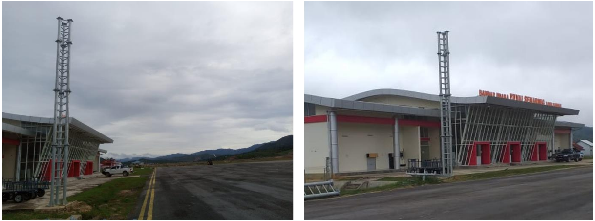
Figure 2: The floodlighting pole
