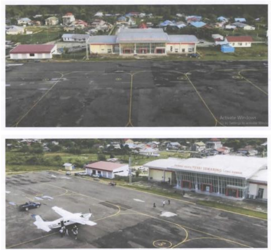
Figure 7: The painted taxiway centerline markings
