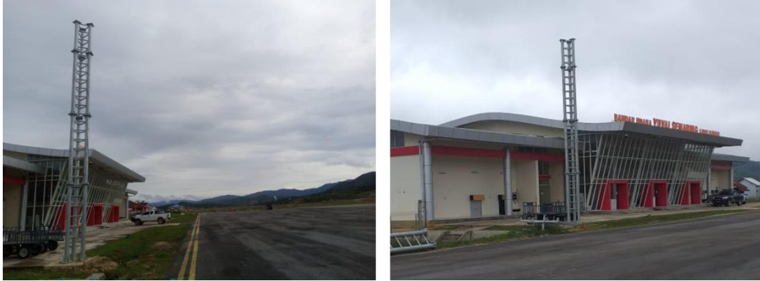
Figure 2: The floodlighting pole
