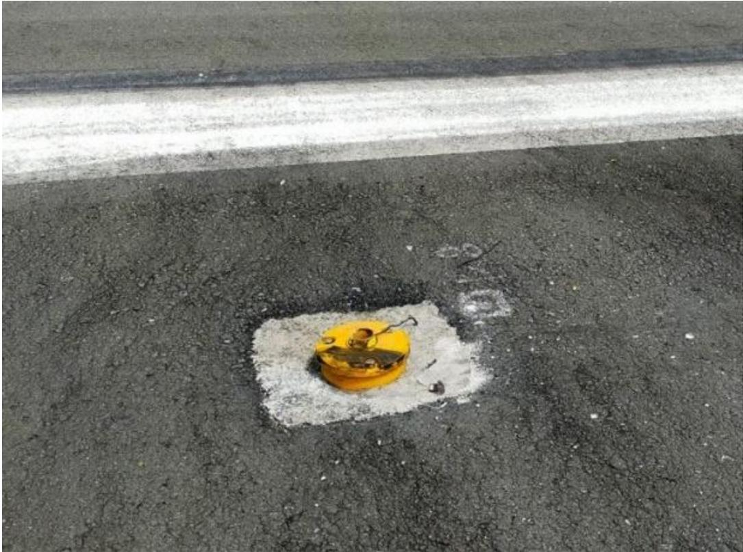
**Figure 2: Damage to runway edge light**
