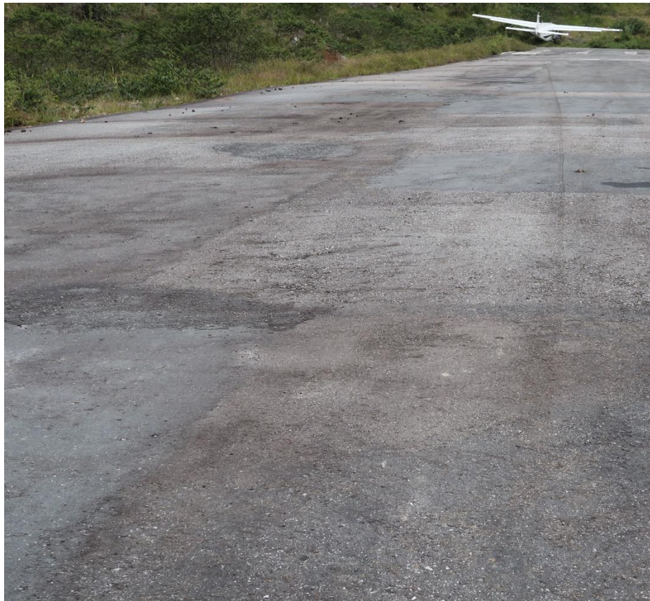
Figure 7: The tire mark found on the runway
