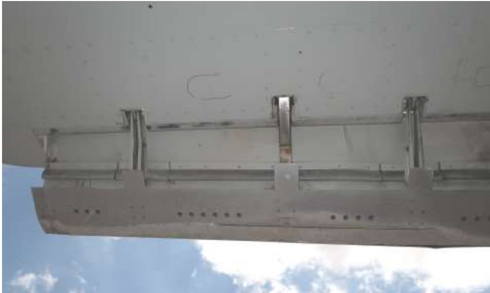
Figure 2 Scratches on the lower surface of the slat leading edge
