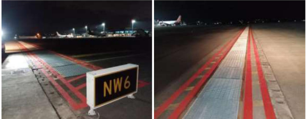
Figure 7: The repaired metal structure and the repainted apron marks
