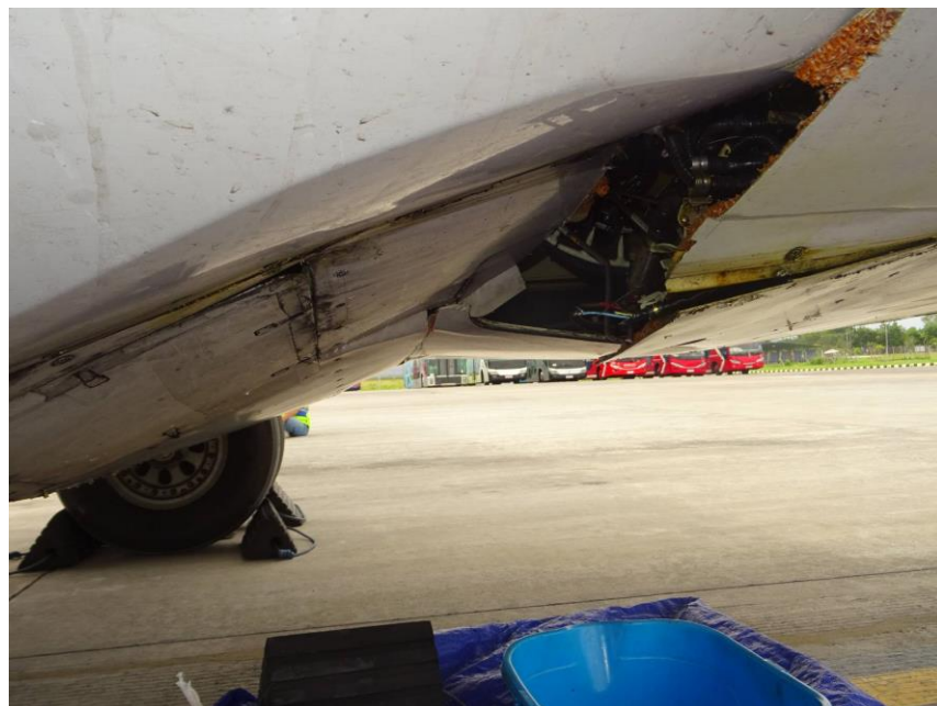
Figure 6: The crack on the lower fuselage aft of the main landing gear compartment
