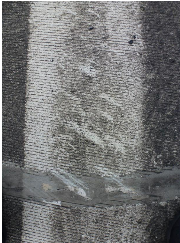
Figure 3: The striation mark on runway surface.
