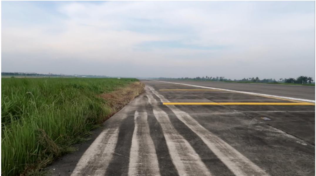
Figure 1: The left main landing gear tire marks before the aircraft out of runway.
