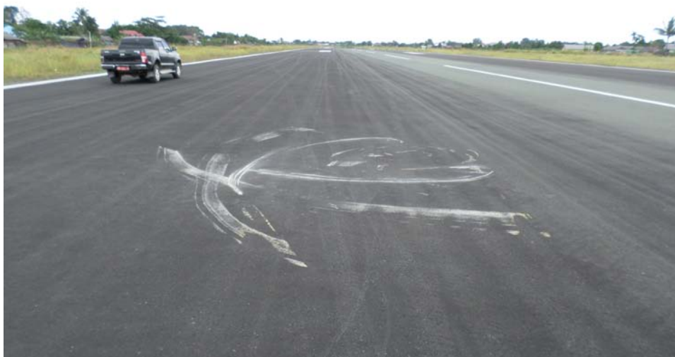
Figure 6: The scratch marks after the helicopter removed
