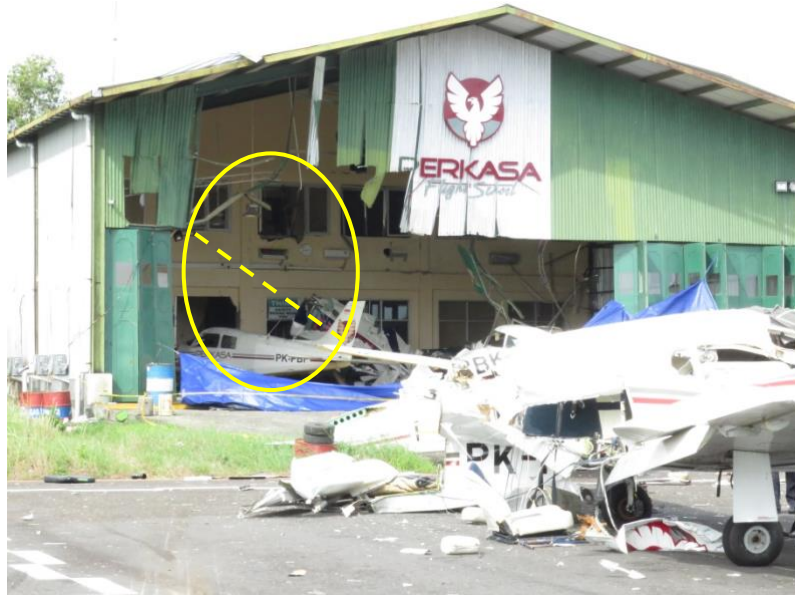
Figure 9: The Damage of the hangar
