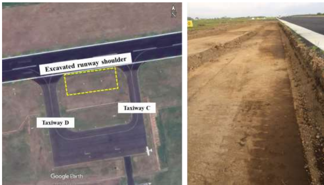
Figure 6: The excavated runway shoulder position and condition
