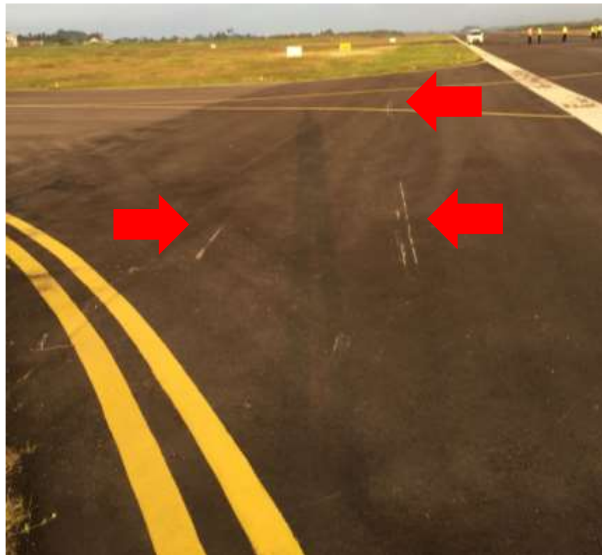
Figure 8: Scratch marks on taxiway D
