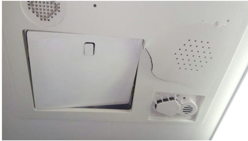
Figure 4: Broken Aft Lavatory Ceiling
