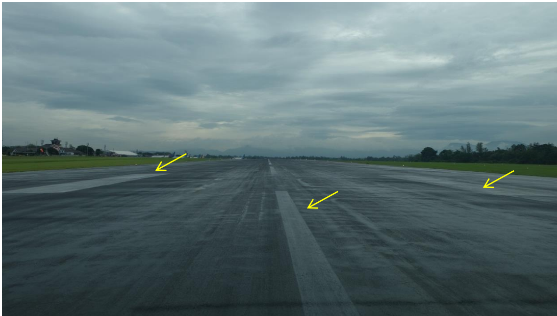
Figure 3: The unclear runway centreline and touchdown bar markings
