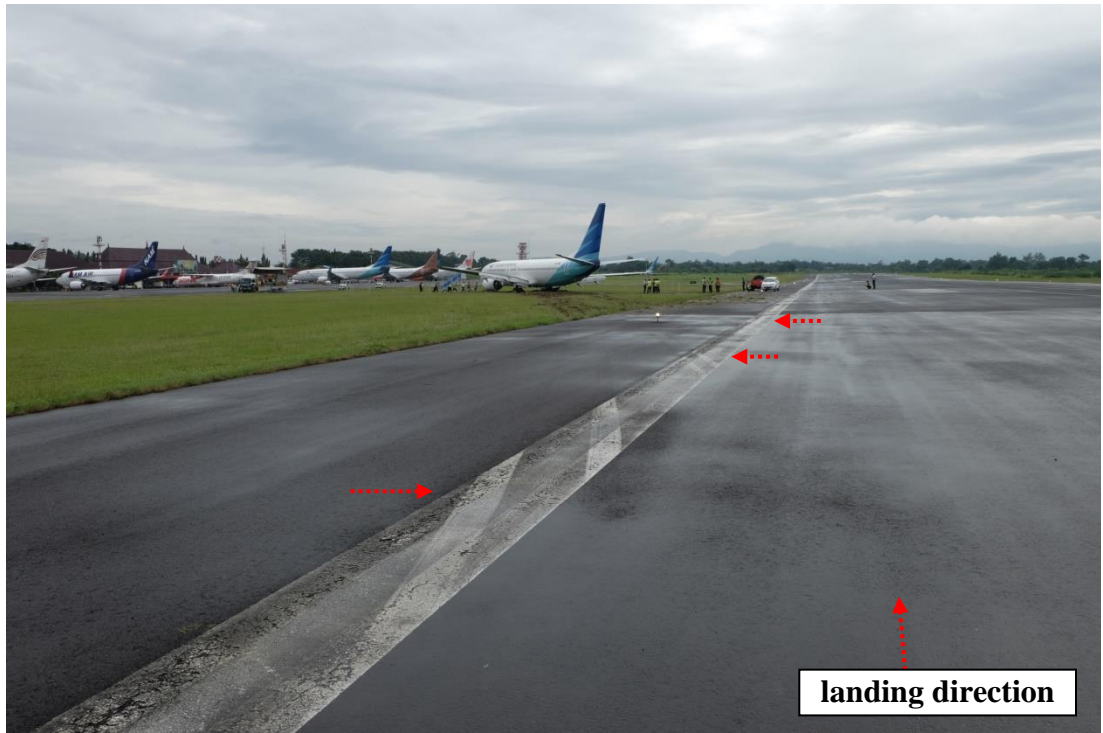
Figure 5: The tire marks on runway and on shoulder
