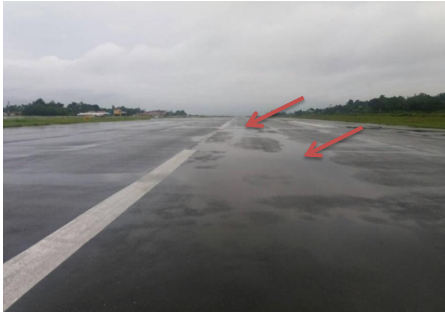
Figure 6: Standing water in the warp runway surface
