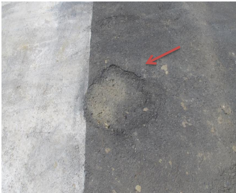
Figure 5: Warp area on the runway surface
