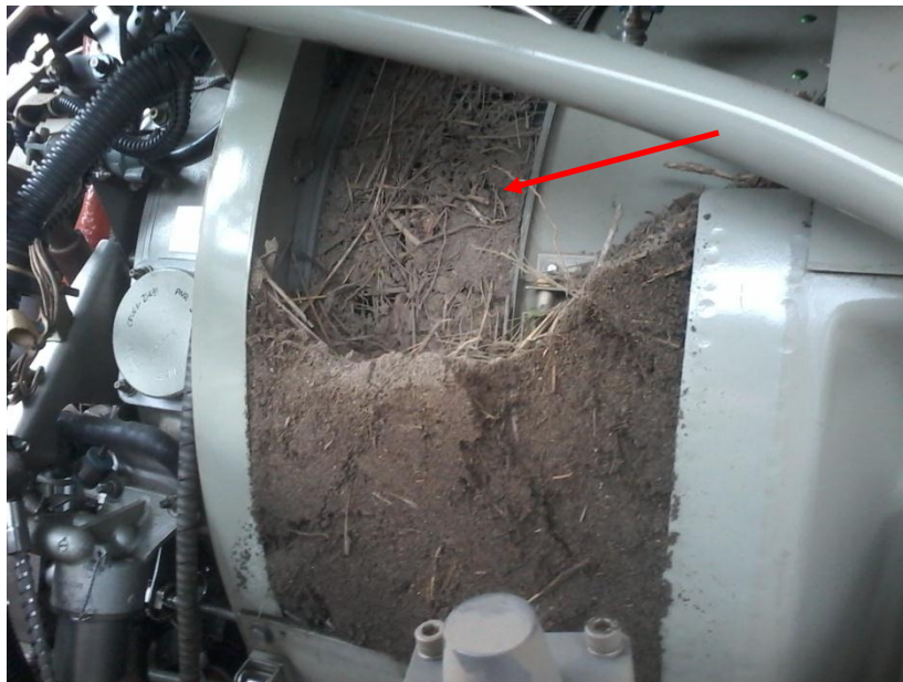
Figure 4: Debris on the screen of the engine compressor air intake
