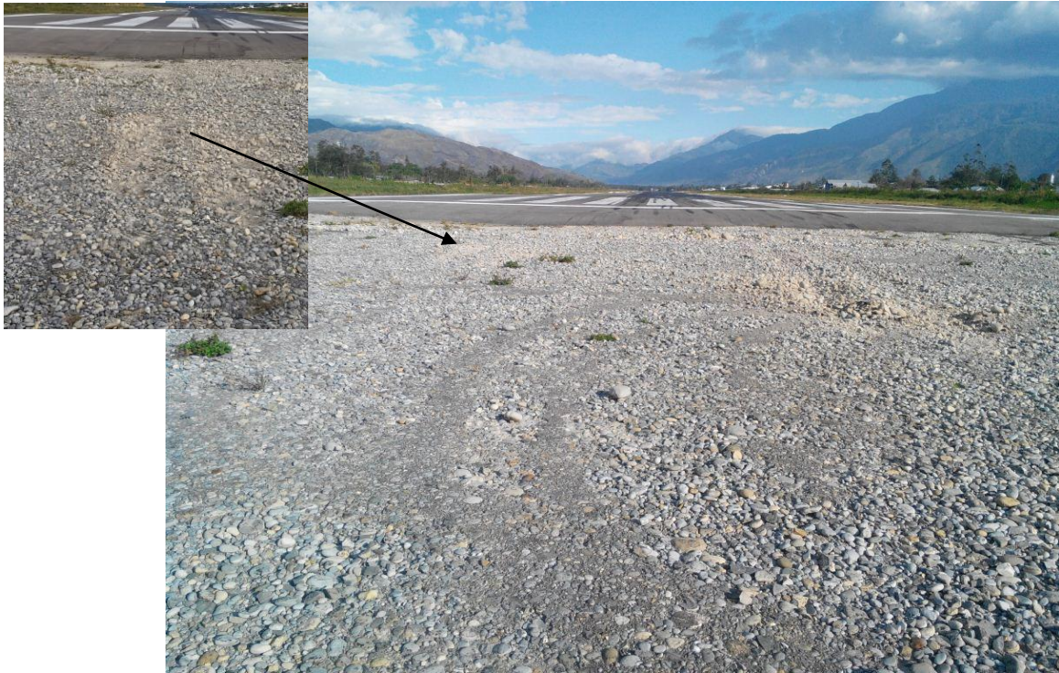
Figure 8: Touchdown mark on the surface before the runway pavement
