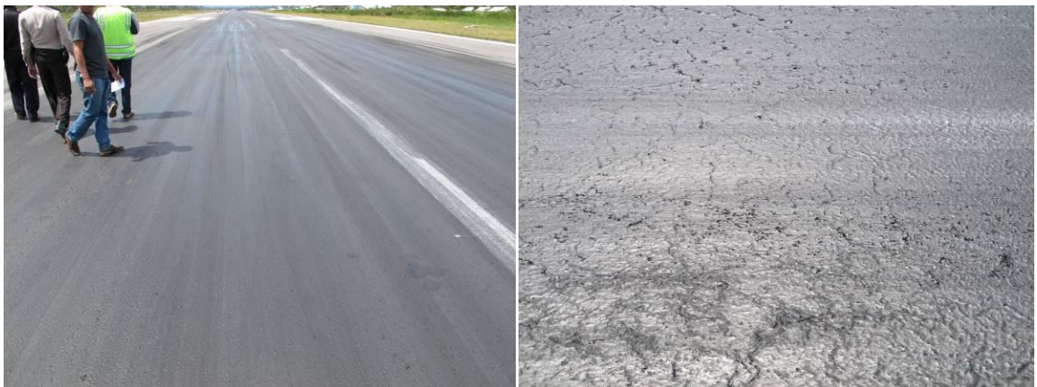
Figure 4: Rubber deposit on runway 15
