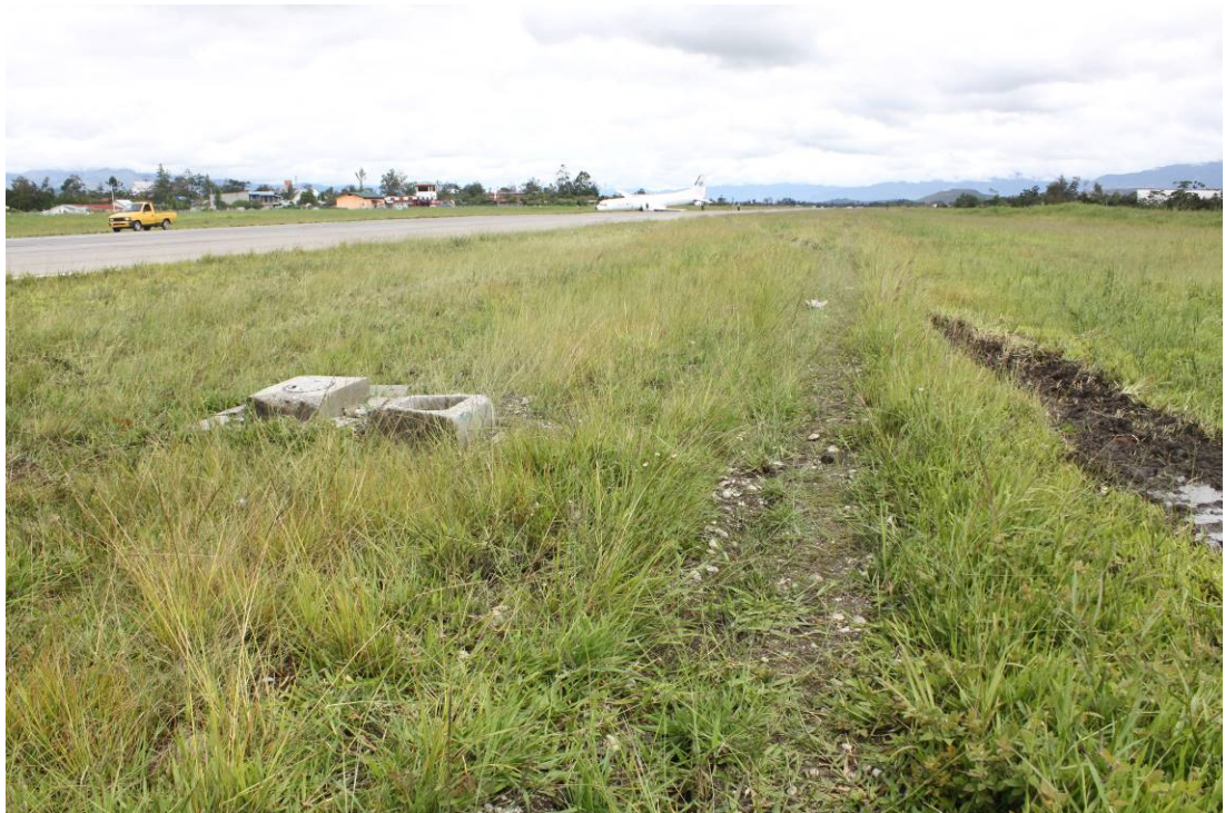
Figure 4: Damage on the runway light hit by the aircraft
