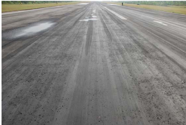
Figure 2: Rubber deposit on the touchdown zone runway 18.
