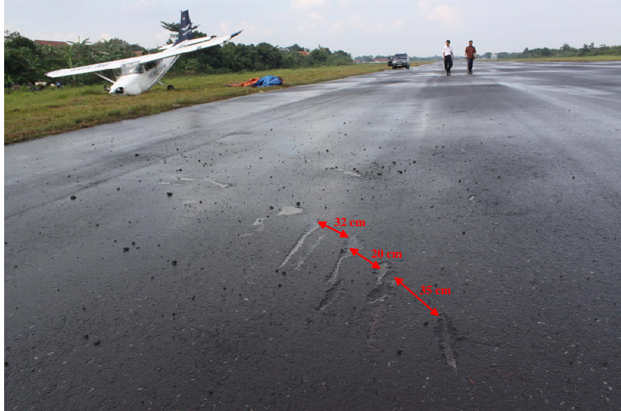
Figure 2: Scratch on the runway surface
