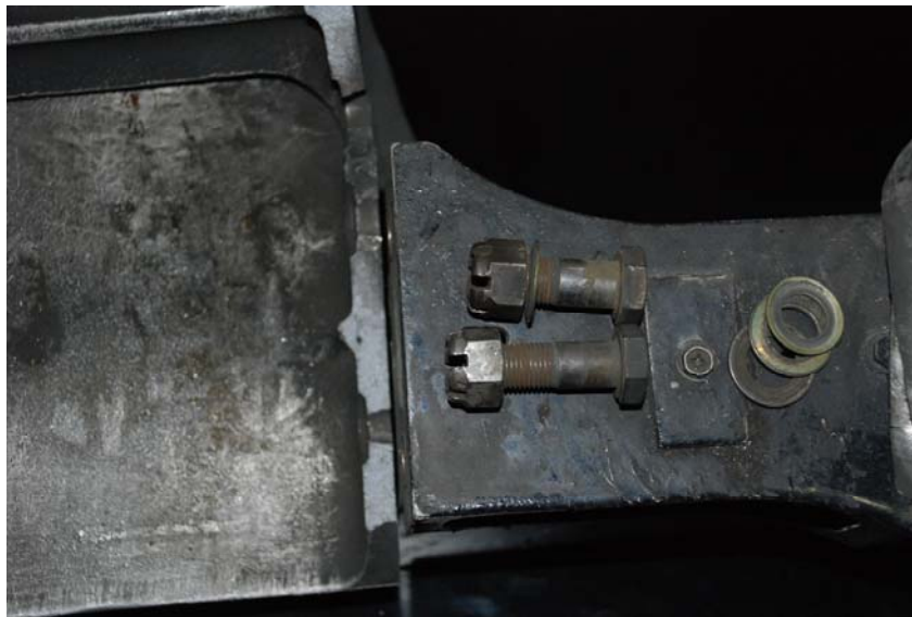
Figure 9: crack area at the right edge
