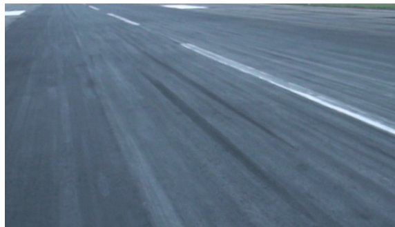
Figure 9: Touch down number 1 and number 2 tire marks
