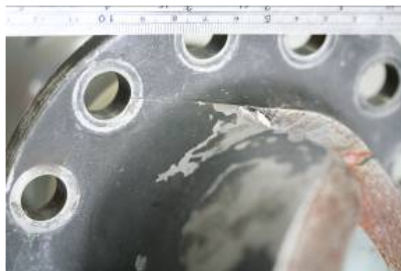
Figure 3: The crack at the hole edge propagated inward
