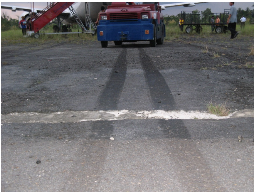
Figure 3: Tire marks on departure end of the runway
