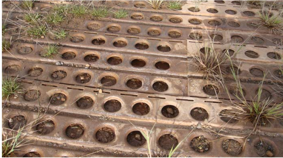
Figure 2: The marsden matting steel plate runway surface
