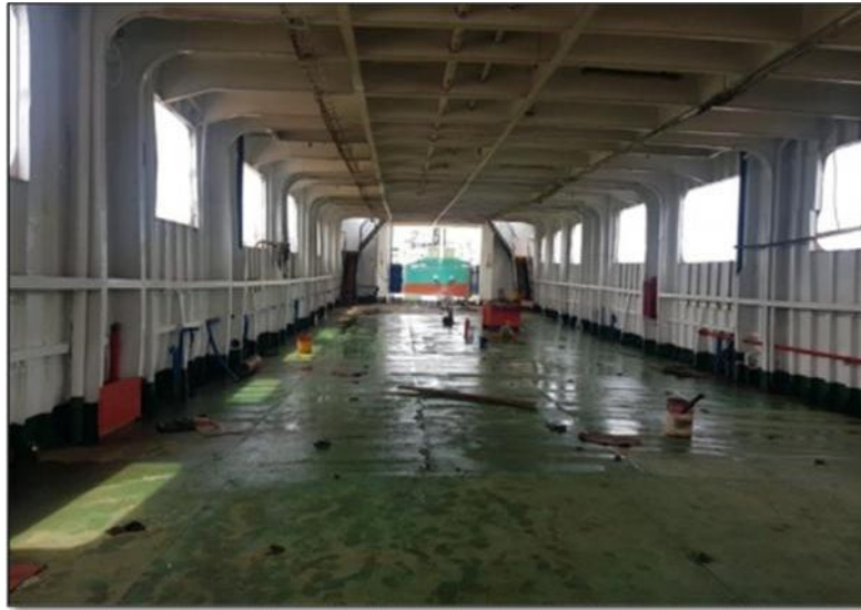
Gambar I-7: Geladak kendaraan (open Ro-Ro space) sumber BKI
