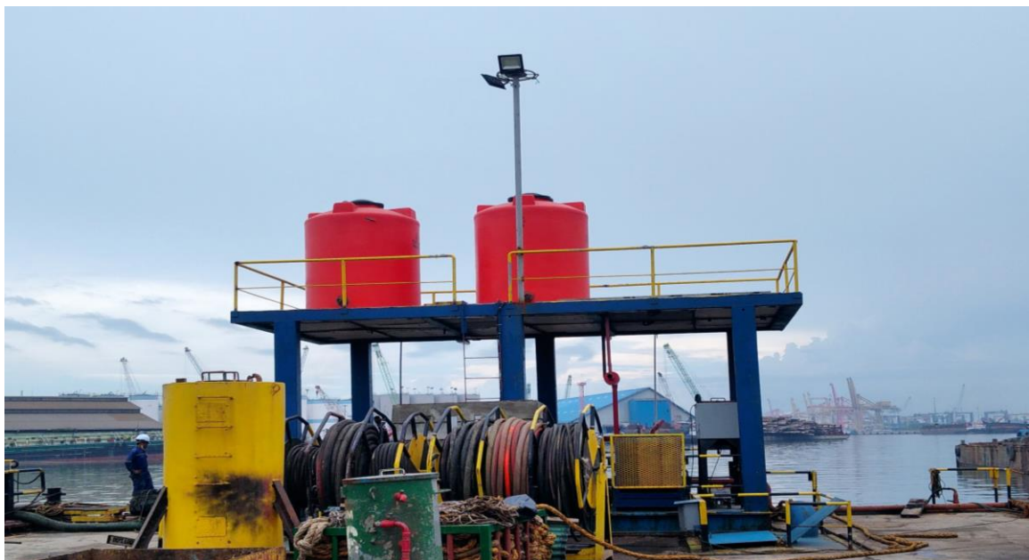
Gambar IV-1: Tangki foam sistem PT WSI
