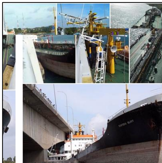
Figure 2: Eastern Glory hit middle pillar of Barelang 2 Bridge
