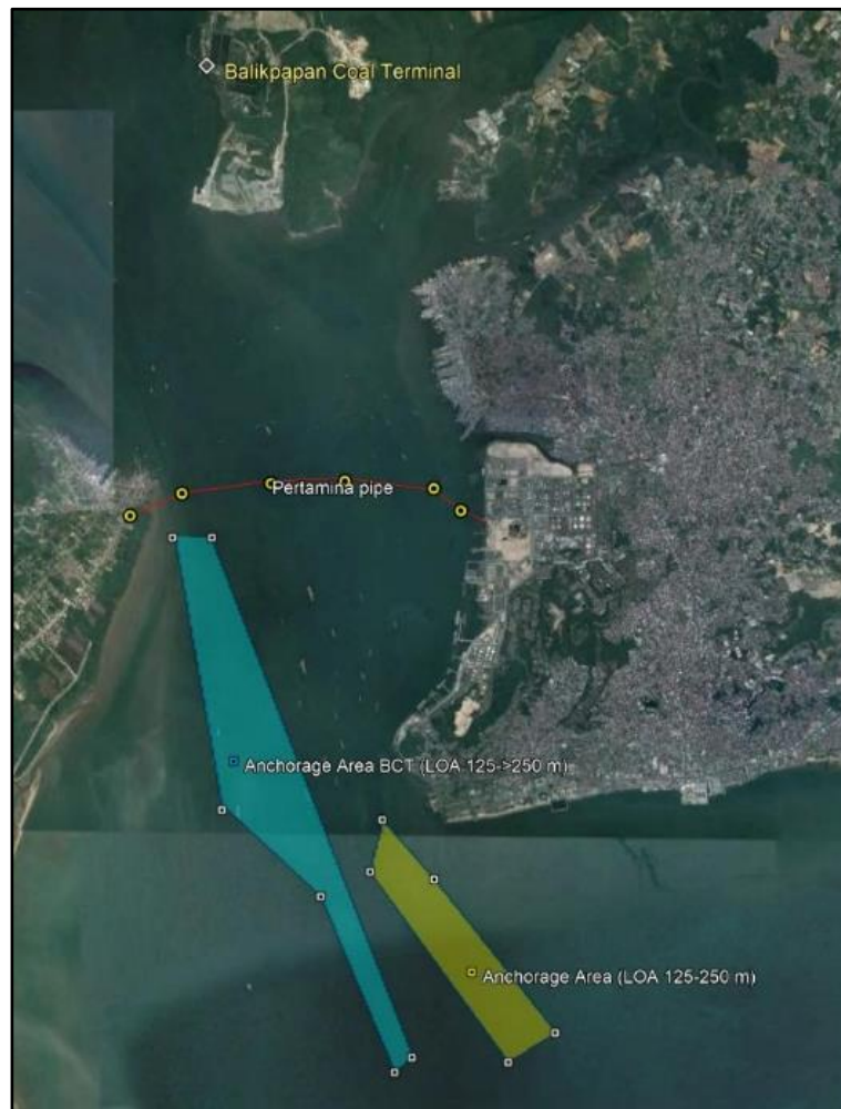
Figure I-34: Anchorage area in Balikpapan (the chart was recreated using Google Earth based on Balikpapan Harbour Master Regulations)
