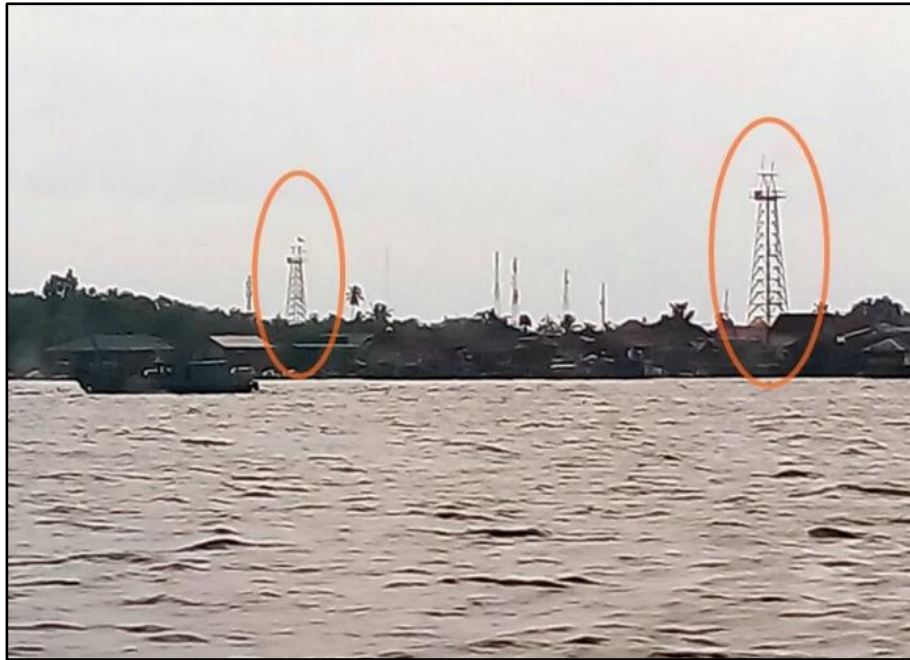
Figure I-32: Towers as subsea pipe markings
