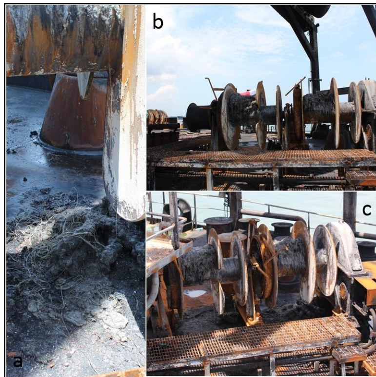
Figure I-11: The burnt windlass on aft port side
