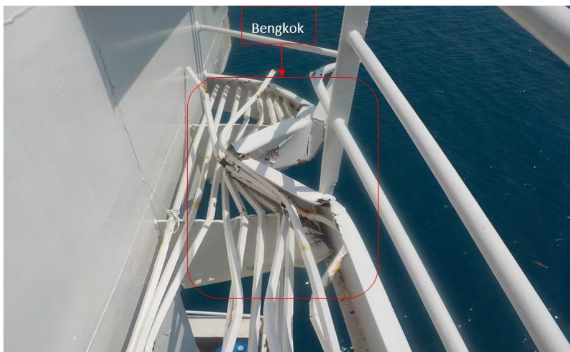
Gambar I-17: Bridge face's catwalk relling.
