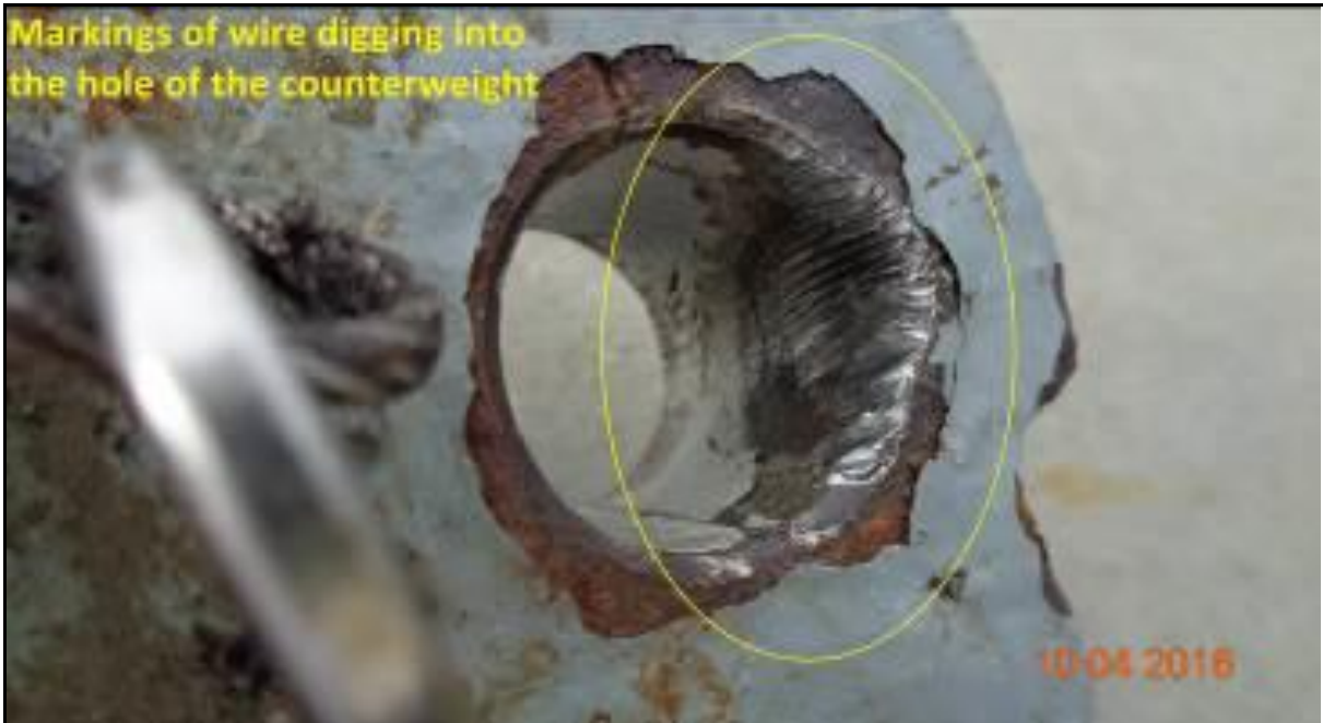
Figure II-2: Condition of the counterweight hole (picture taken from company investigation report)
