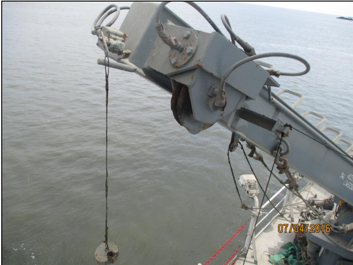
Figure I-17: Hoist limit switch
