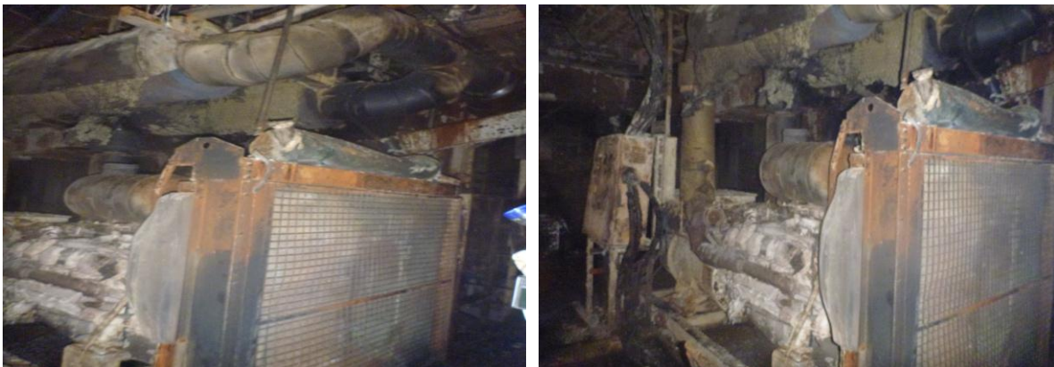
Gambar I-3: Mesin emergency generator menggunakan radiator (Non Marine Standard)
