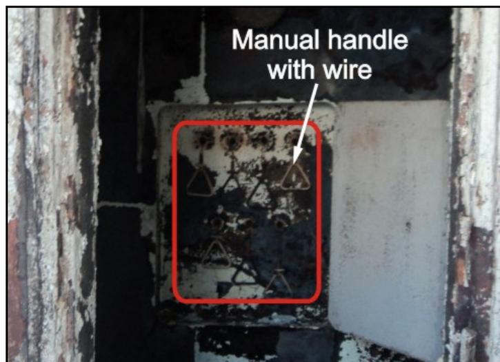
Gambar I-10: Panel emergency quick closing valve
