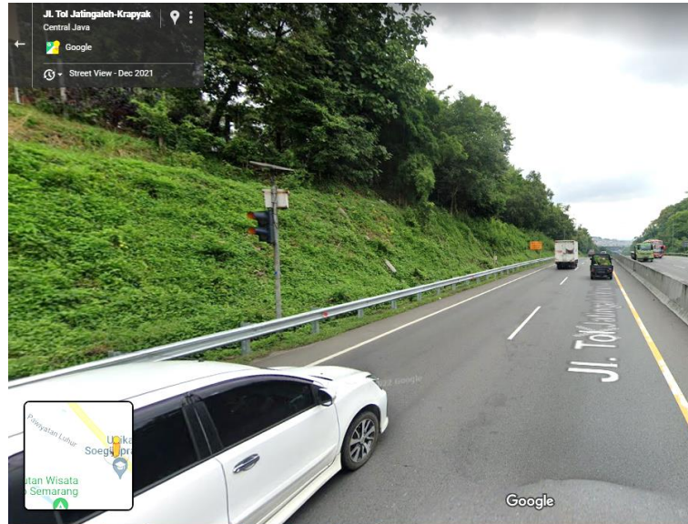
Gambar 10. Lampu Peringatan ( Warning Light ) solar cell
