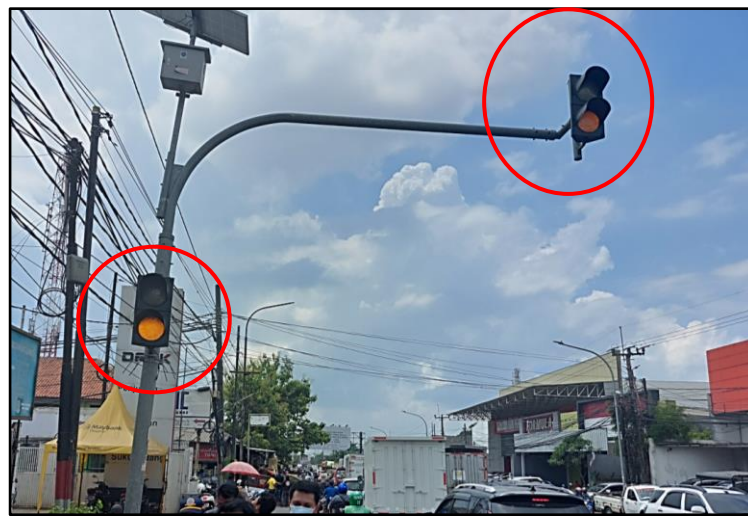
Gambar 9. lampu peringatan ( solar cell warning light )
