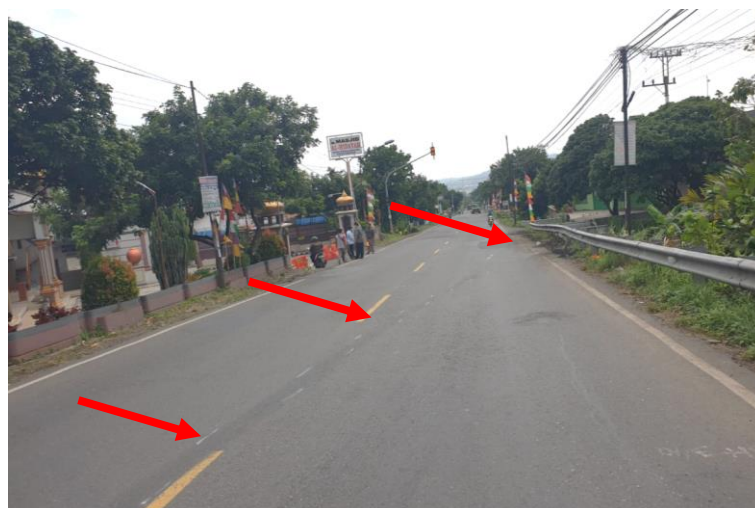
Gambar 15. Skid marks ban dump truck menuju guardrail jalur lawan arah
