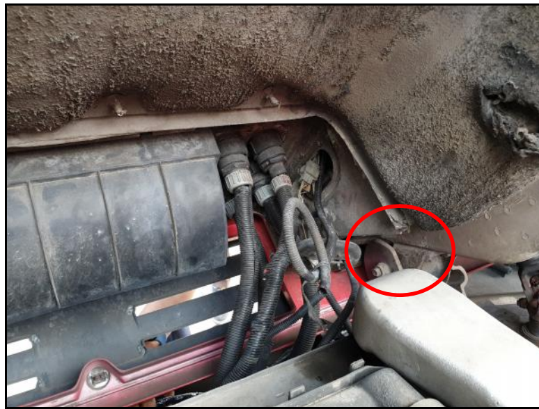
Gambar 10. Kondisi cabin mounting aus
