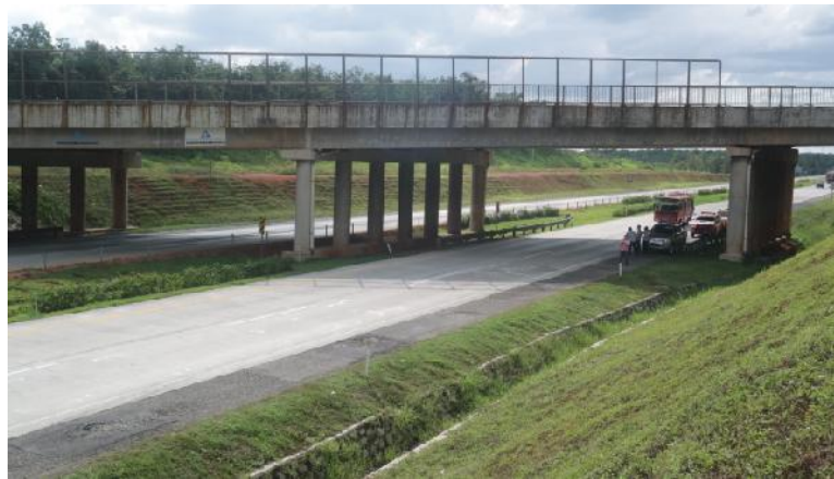
Gambar 11. Jalan Tol Cipali KM 78+500 A
