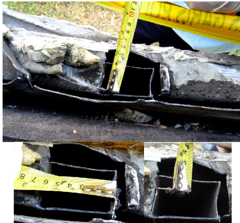
Gambar 8. Rangka dinding besi hollow ukuran 40x60x1 mm
