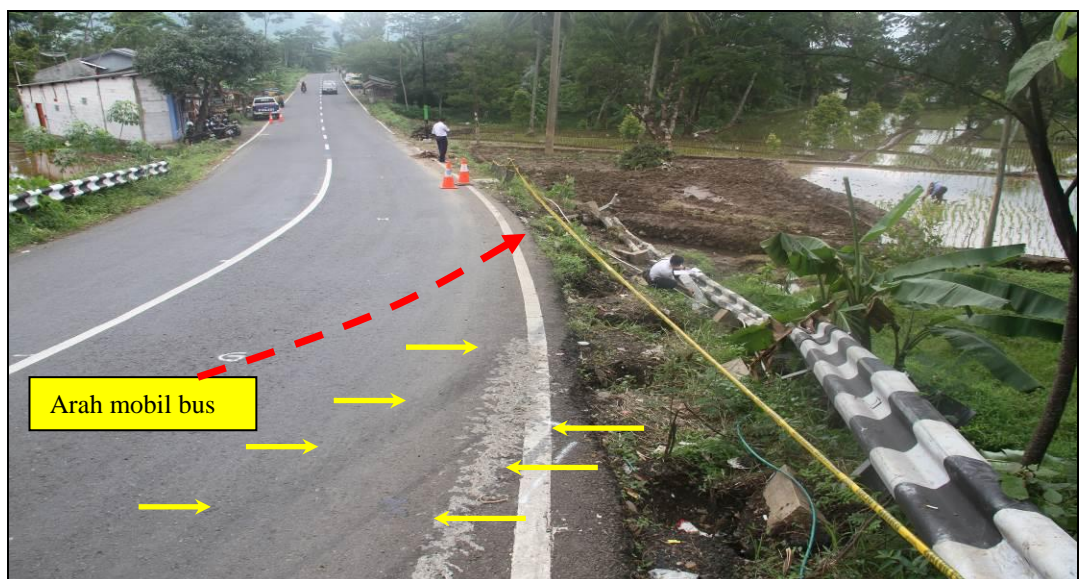
Gambar 9. Skidmark mobil bus.
